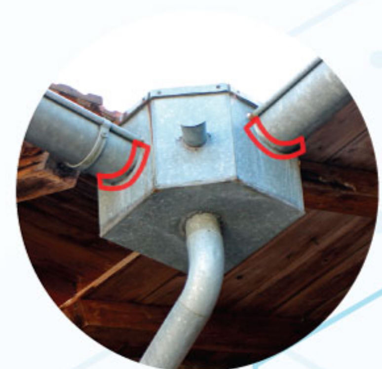
SEALING GUTTER LEAKS
