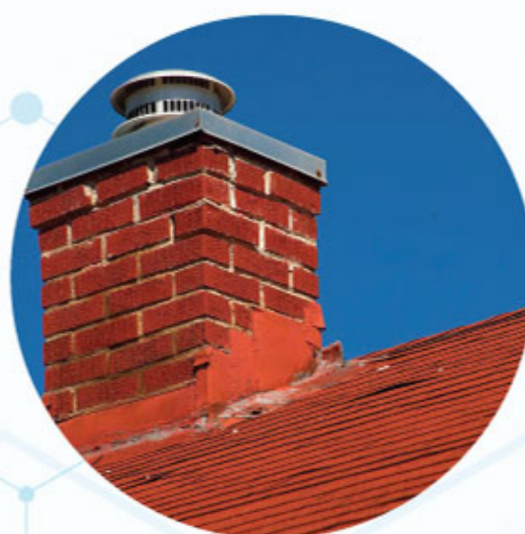
SEALING AROUND CHIMNEY
