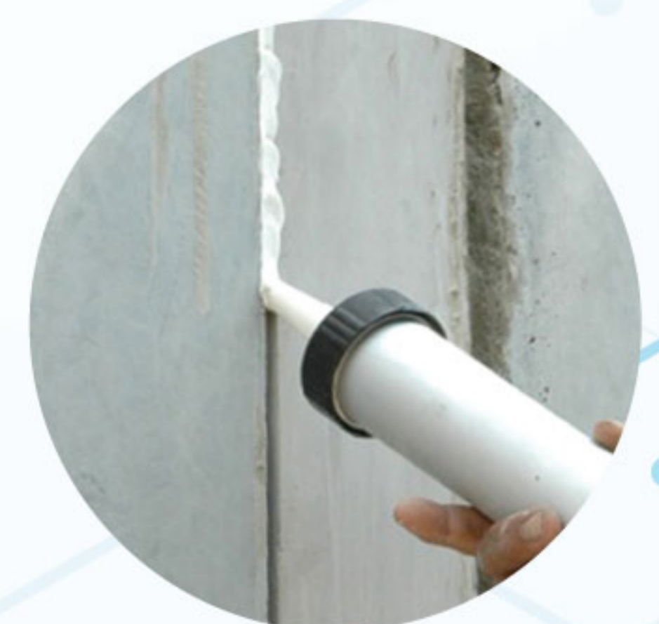
PRECAST WALL PANEL JOINT
