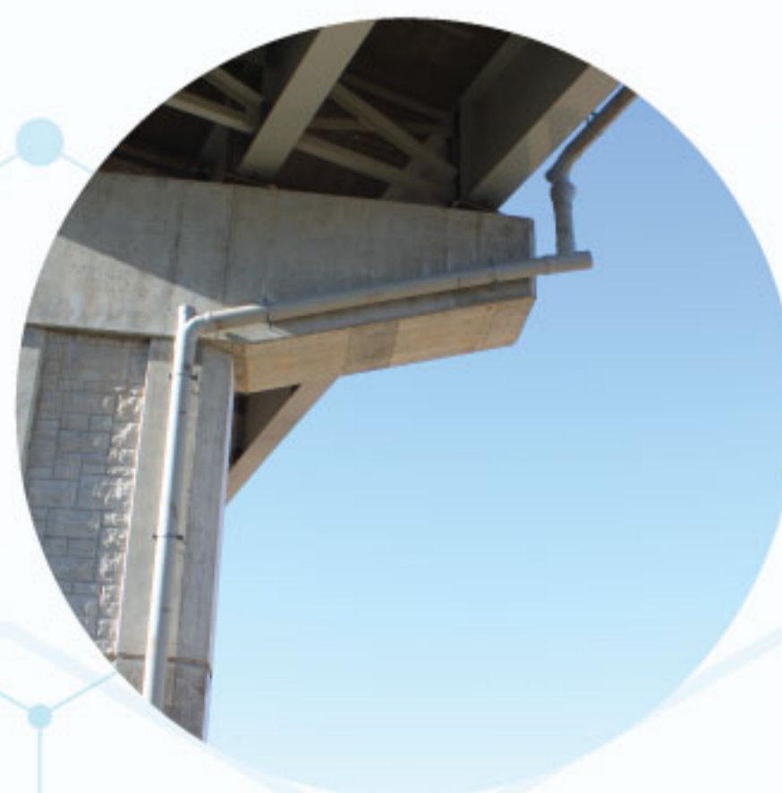
BRIDGE DECK DRAIN
